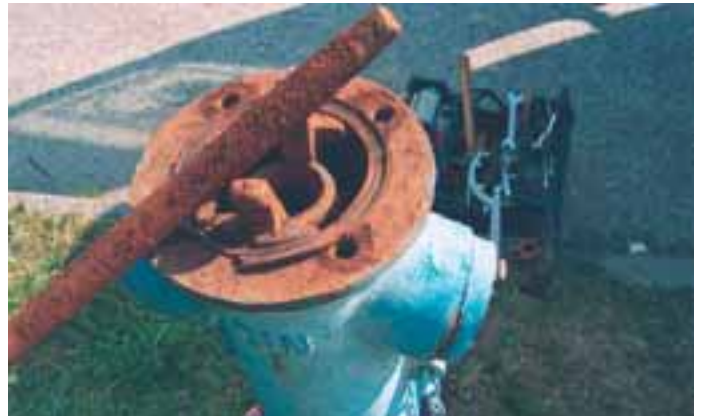
Hydrantenservice (Tausch "Innereien")
